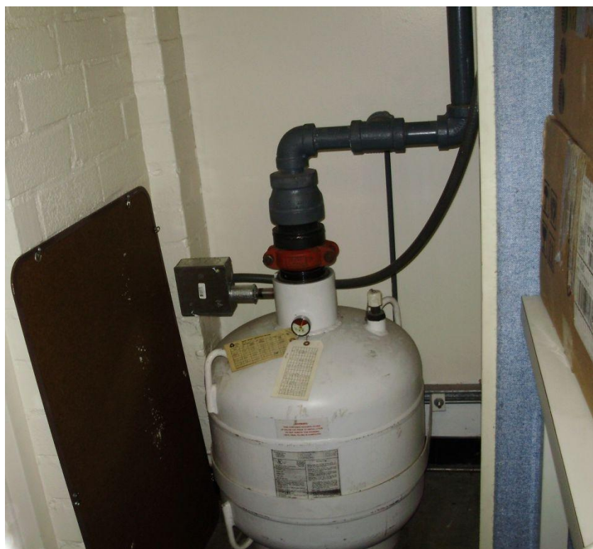
Figure 3-1. Typical Halon 1301 Total Flooding System
